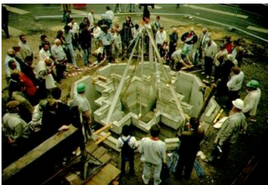
Fig. 7 Completion of installation of inverted fountain
